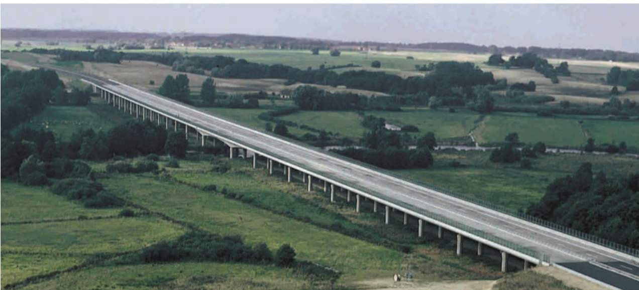
Figure 7.36 - Instead of building an embankment, the motorway A20 in northern Germany was built on pillars. This low viaduct preserves the floodplain and marshes below. (Photo by DEGES)
